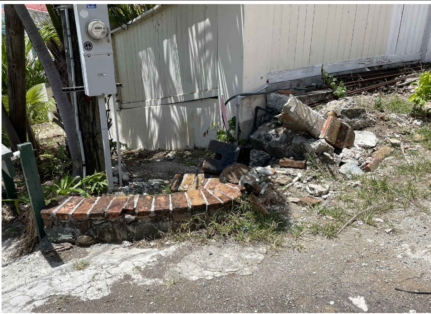
A LOW MASONRY CURB TO BE REPAIRED
