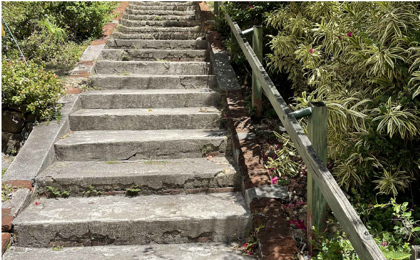
B SAMPLE AREA FOR MORTAR LAYER REMOVAL TO RESTORE NATURAL BRICK APPEARANCE
